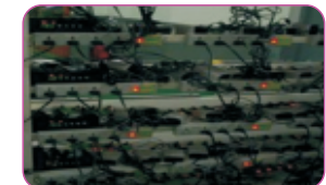
Aging Test Room
